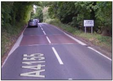
EXISTING COLOURED ROAD NARROWING TO BE REINSTATED TO ORIGINAL CONDITIONS PER IMAGE
